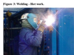
Figure 3: Welding, hot work.
